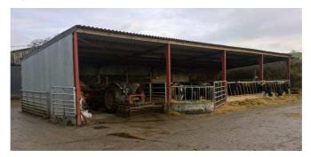
H) Steel portal framed cubicle building, 120' x 36' providing cubicle housing for 60, fibre cement roof cladding, mass concrete walls to 1/3 height and spaceboarding above to sides and rear with feed barrier to front under cantilever overhang. Feeding/scraping passage adjacent to sheeted door giving access to slurry store. Internal strip lighting, water supply with concrete base and apron. Full height sheeted doors to both gable ends.
